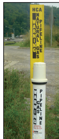
5. HCA marker and cathodic protection test station
