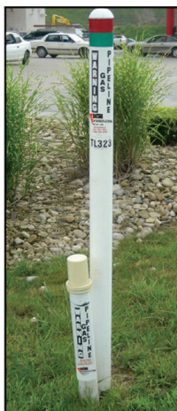
2. Linemarker and cathodic protection test station
